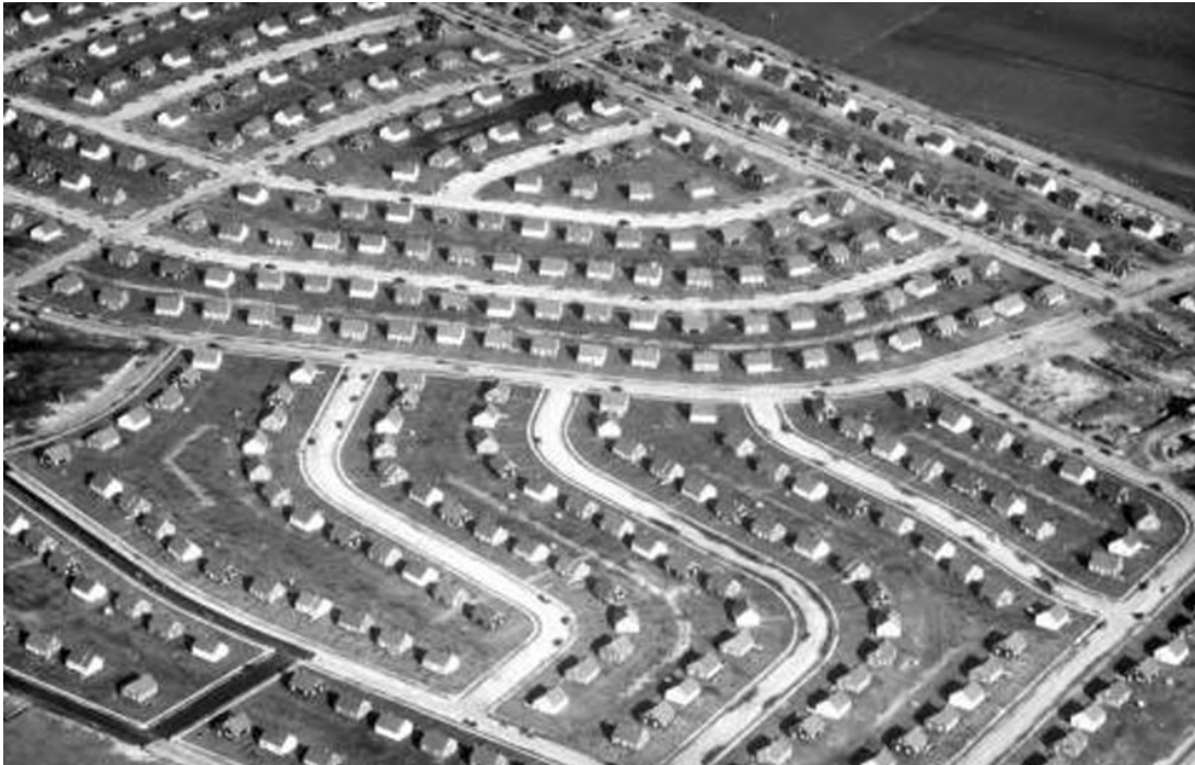
Aerial View of Tract Housing, Levittown, NY, 1949
