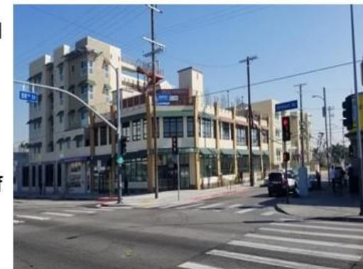
*Photos of the first HHH project that completed construction, 88th & Vermont, located at 8707-27 S. Menlo.
